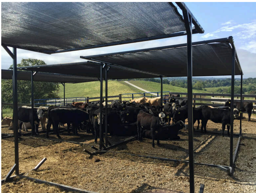
Shade Structure Eden Shale Farm Owenton, KY
